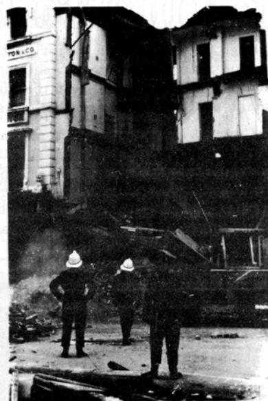
Firemen at the scene of the collapse.
