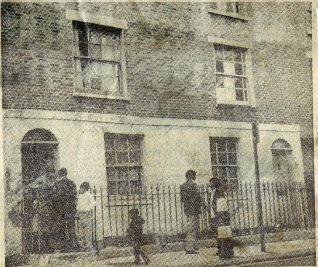
The two condemned properties where Bengali families are crowded in one family to a room.
