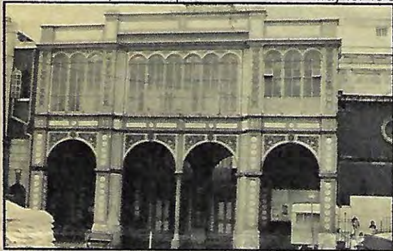
Floral Hall, Covent Garden Included in plans for Opera House extension, although recently listed
