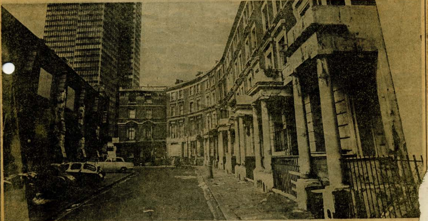
Crumbling facades in Tolmers Square—soon to be replaced by another Euston Road tower block?
